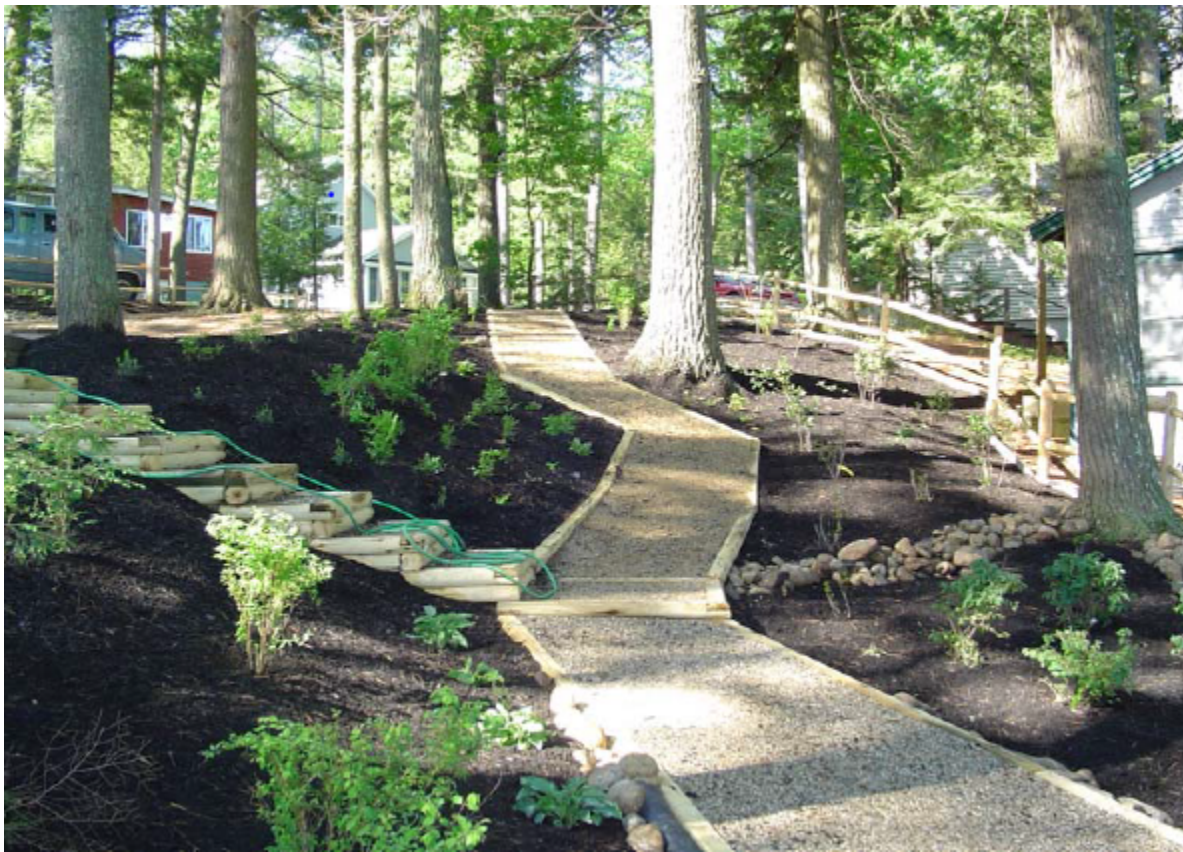
Photo from a Forest Lake property addressed in the early 2000s. Improvement practices installed included infiltration steps, defined walking path, native plants, and erosion control mulch.
