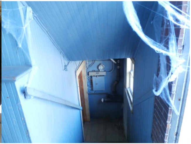
Figure 2: Stairwell to Basement
