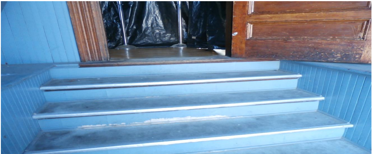
Figure 3: Stairs Front Entry
