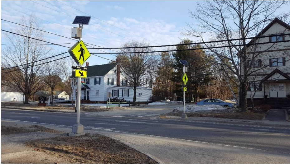
FIGURE 4: NEW CROSSWALK ON RTE 26 BETWEEN FIDDLEHEAD CENTER AND GRAY PARK IMPROVES WALKABILITY AND SAFETY FOR STUDENTS.
