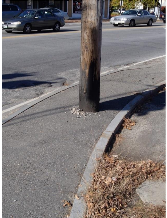
FIGURE 10: SIDEWALK IN FRONT OF MANNY'S MOTORS WITH TELEPHONE POLE.
