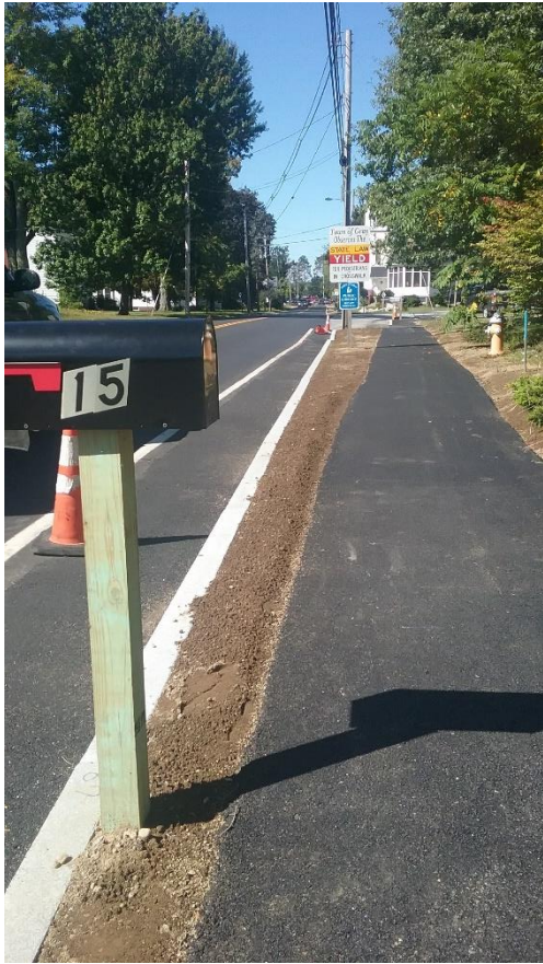
FIGURE 5: BROWN STREET SIDEWALK RECONSTRUCTION, LOOKING WEST TOWARD VILLAGE
