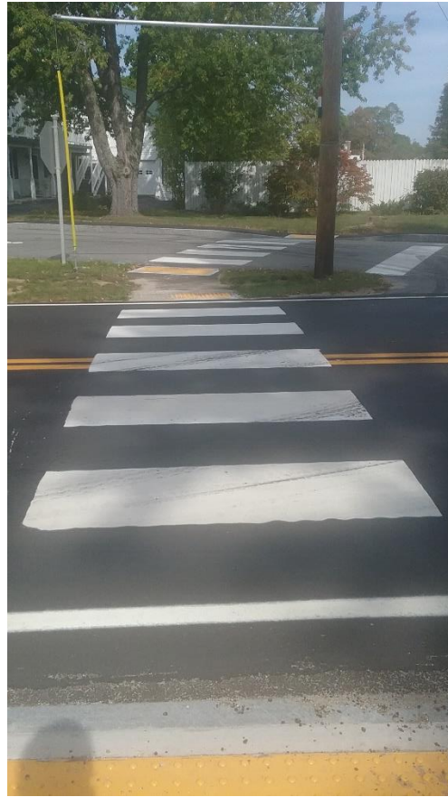
FIGURE 6: NEW CROSSWALK AND SAFETY ISLAND, LOOKING NORTH ACROSS YARMOUTH RD. AND BROWN STREET.
